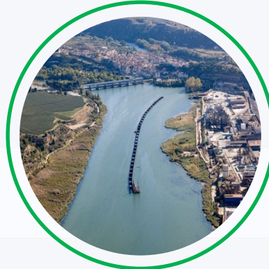
Decontamination of Flix Reservoir - Spain
