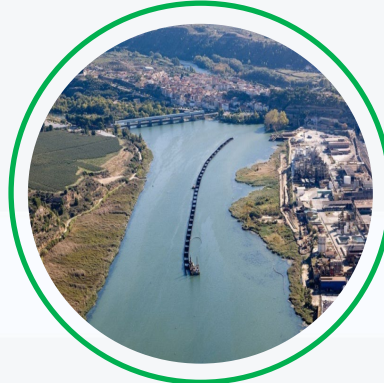
Decontamination of Flix Reservoir - Spain
