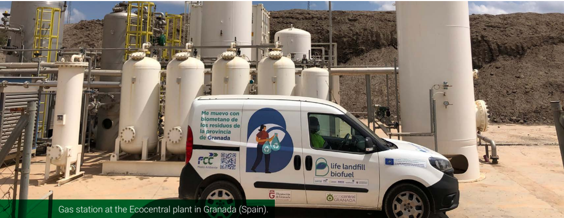
Gas station at the EcoCentral plant in Granada (Spain).
