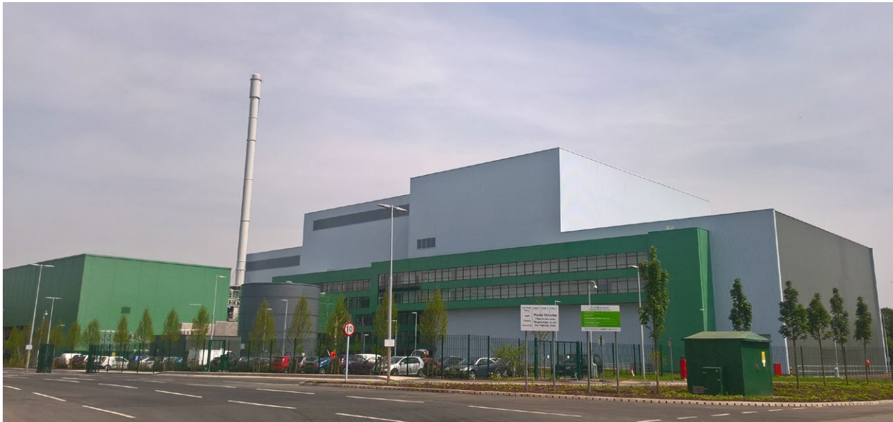
EnviRecover Energy Recovery Plant in Hereford and Worcester (United Kingdom).
