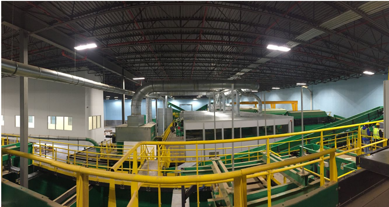
Recycling plant in Dallas (Texas, USA).
